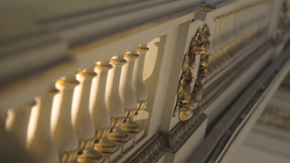
Balustrade - Salon Guillaume Dupré - Quai de Conti Railing in the Guillaume Dupré room at the Quai de Conti
